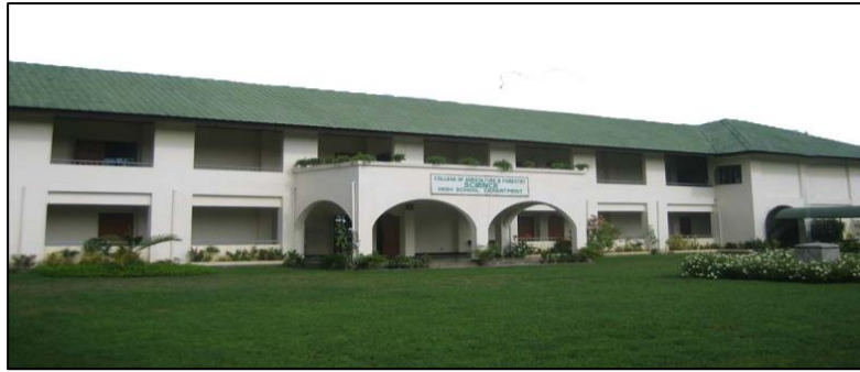
Figure 7. An image showing the Laboratory High School Batac Campus https://m.facebook.com/pg/MMSULHSBATAC/photos/?ref=page_internal
