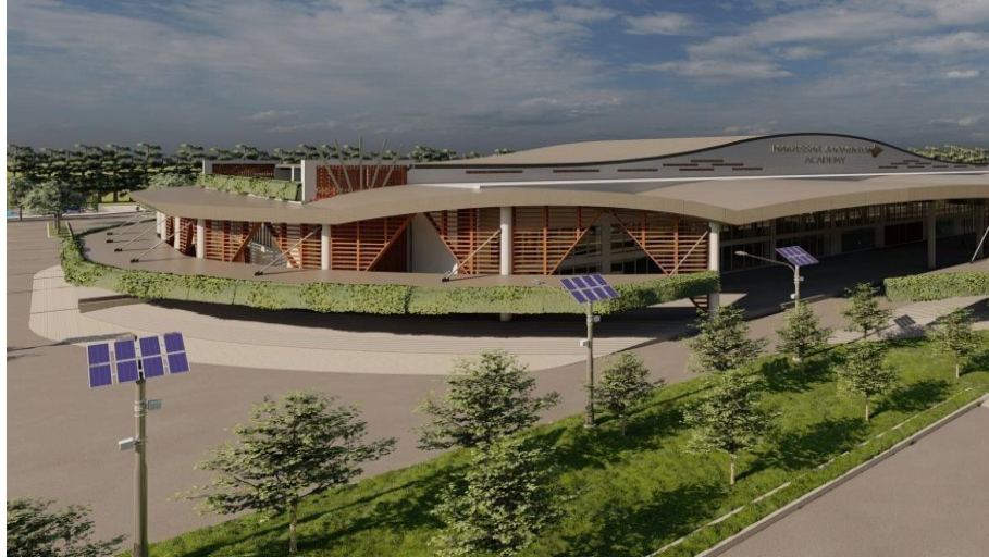
Gambar 4: Lampu Jalan Solar Panel
