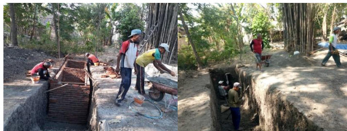
Figure 9. Process for making wastewater shelter tank
