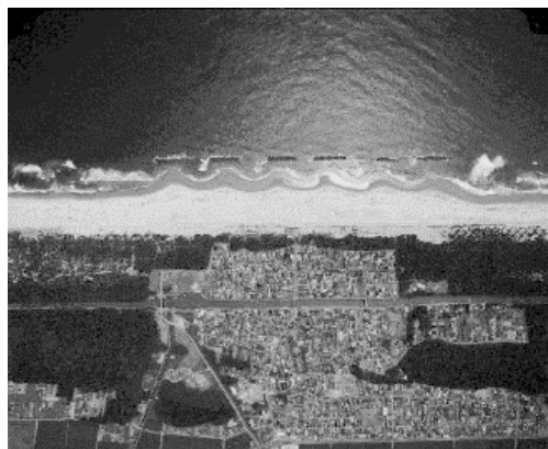
Figure 2. Detached Breakwater in Sendai Coast, Japan (Source: Tohoku univ. 2008)
