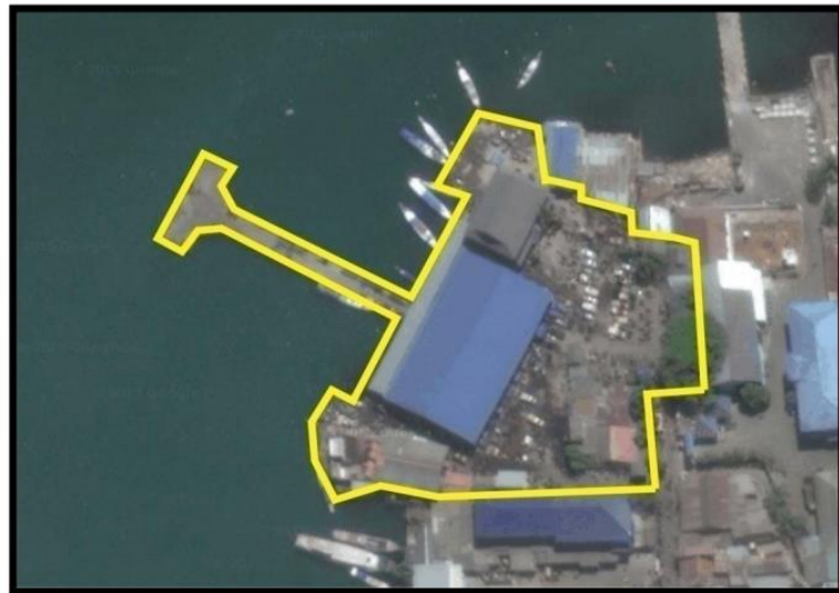
Figure 2. Paotere Fish Landing Station of Makassar (Source: UPTD Paotere Makassar, 2019)
