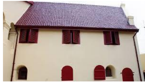
Gambar 12. Jendela Benteng Fort Rotterdam Sumber: https://catperku.com/benteng-fort-rotterdam-makassar
